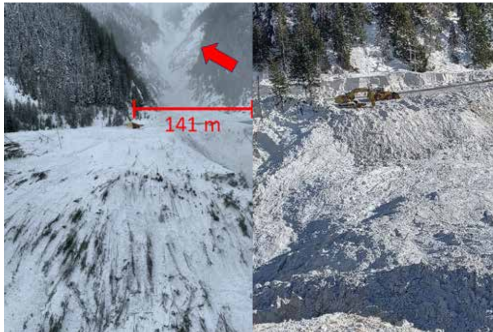
FIG. 6: THE AFTERMATH IN JACK MACDONALD. THE LEFT IMAGE SHOWS SOME OF THE 3.1 HECTARES OF FOREST DESTROYED BY THE AVALANCHE. THE RED ARROW POINTS TOWARDS ANOTHER 2.3 HECTARES DESTROYED IN THE LOWER TRACK AS THE AVALANCHE SUPERELEVATED. FOR SCALE, THE SNOW SHED IS 141M LONG. THE RIGHT IMAGE SHOWS MACHINERY CLEARING OVER FIVE METRES OF SNOW FROM THE CP RAILWAY LINE ACROSS THE RIVER. DEBRIS IN THE ILLECILLEWAET RIVER WAS ESTIMATED AT 25-30 M DEEP.
