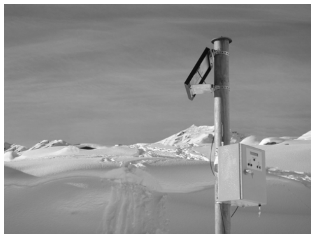
Mammut’s European avalanche training centre features a portable and a fixed beacon control unit. The fixed unit, shown above, is powered by solar cells.
