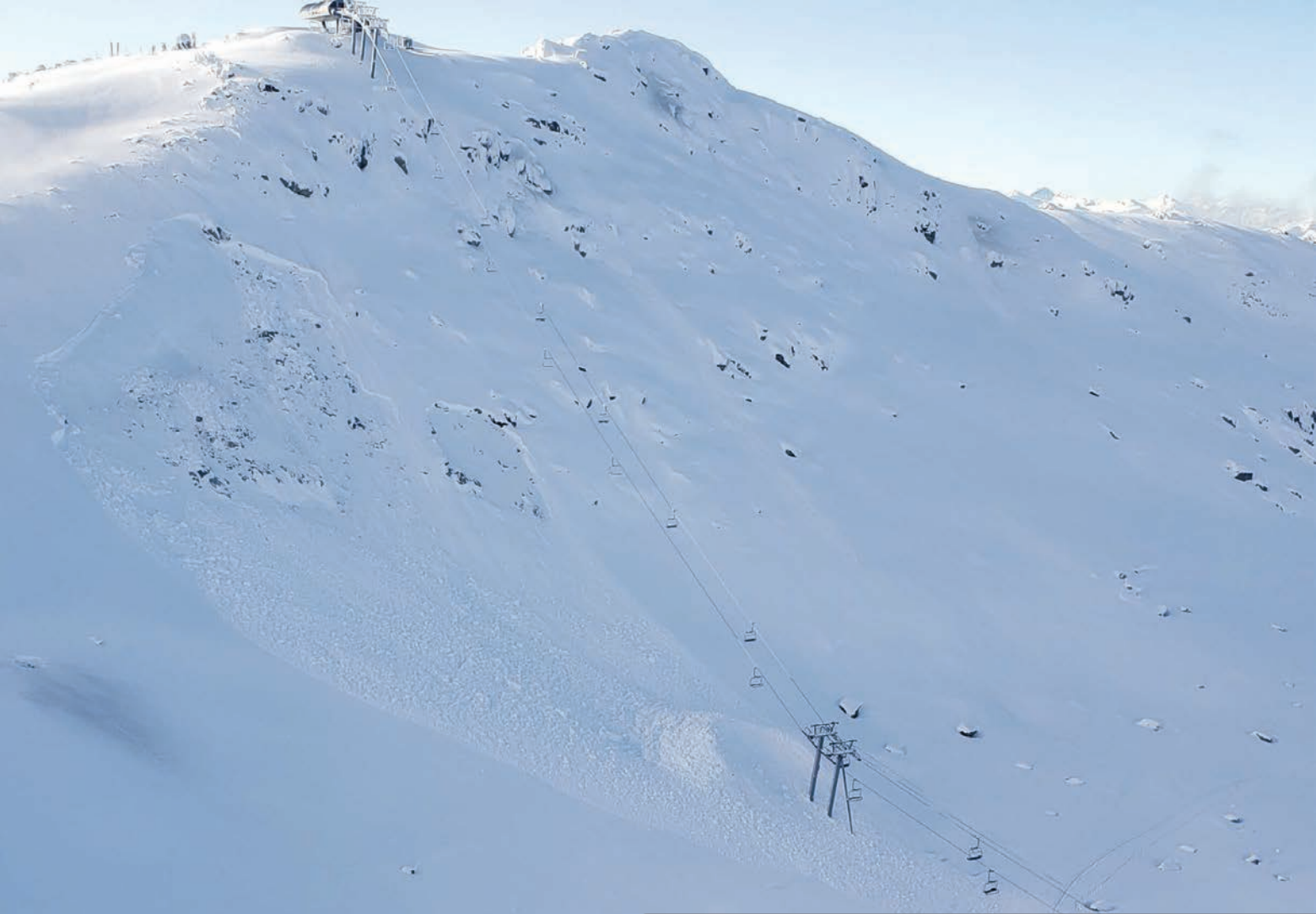
A SIZE THREE AVALANCHE IS DEFLECTED AWAY FROM ONE OF THE TOWERS ON THE SYMPHONY CHAIR BY AN EARTH BERM. IT WAS TRIGGERED DURING A HELICOPTER CONTROL MISSION ON DEC. 21, 2019. // TIM HAGGERTY
