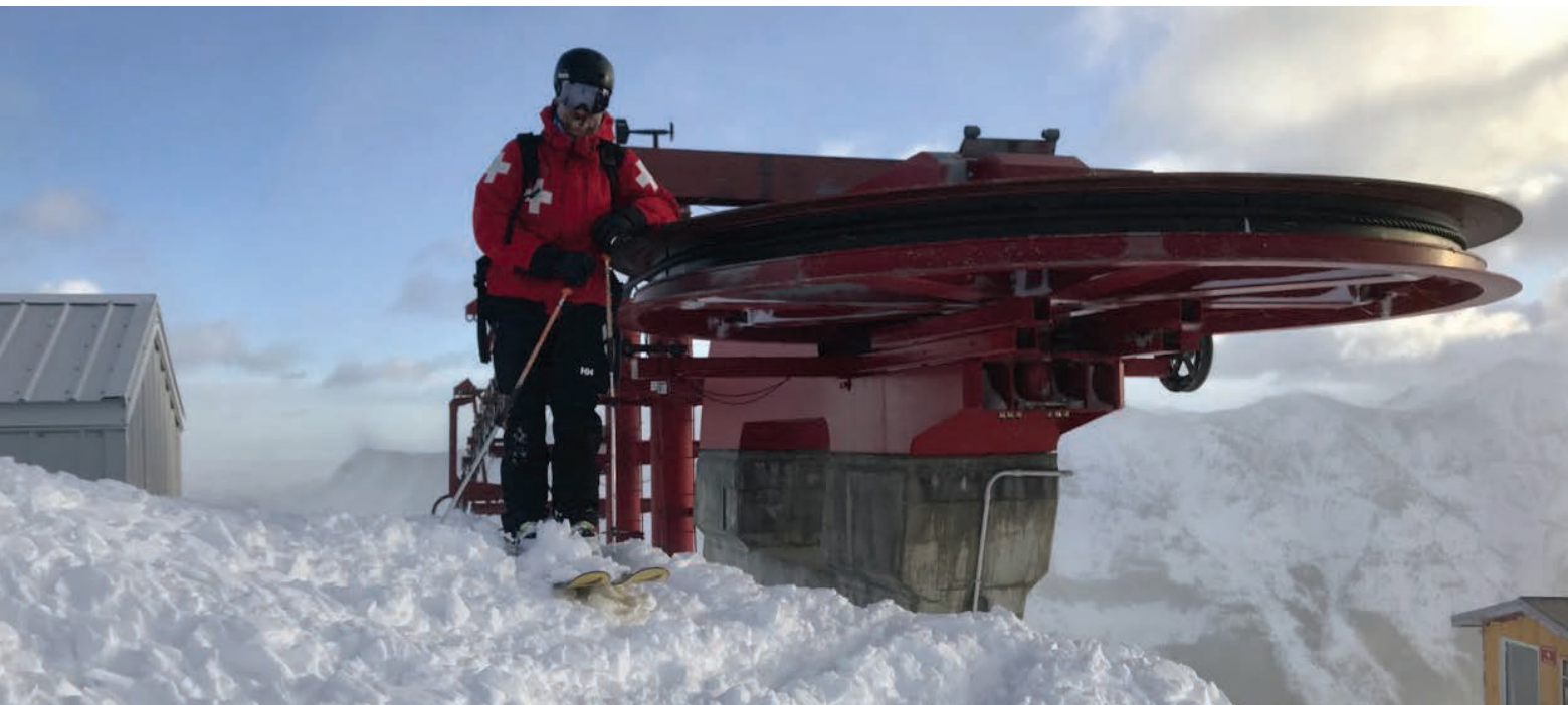
MITCH SULIAK STANDS ON TOP OF AVALANCHE DEBRIS PRODUCED BY EXPLOSIVES CONTROL WORK ON RED CHAIR DRIFT. THE PHOTO DEMONSTRATES THE FEATURE’S POTENTIAL TO IMPACT LIFT INFRASTRUCTURE. // NATHAN PINCHAK
