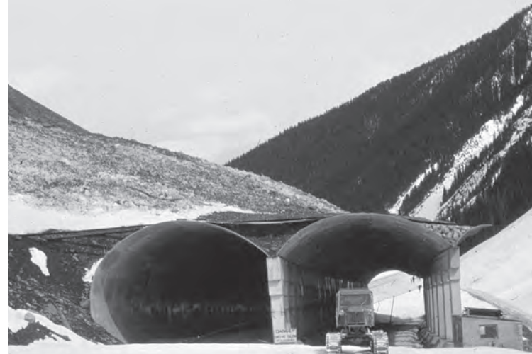
FIG. 2: PIONEER (A.K.A. SPUTNIK 1) SNOWSHED UNDER CONSTRUCTION IN 1961 // REVELSTOKE MUSEUM AND ARCHIVES PSS. 67
