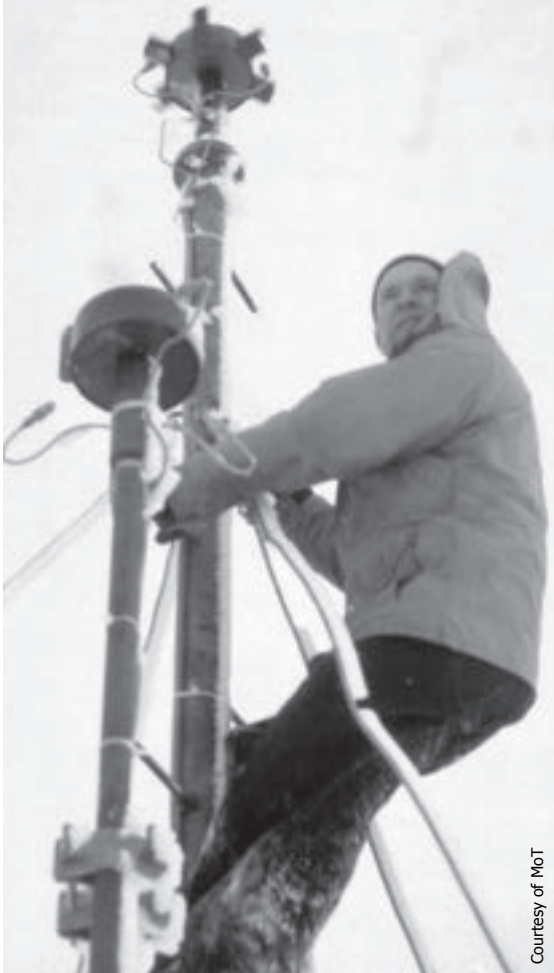
Mike Zylich tuning up the Kiwi Squirt de-icing system at an early Highways Remote Station.
