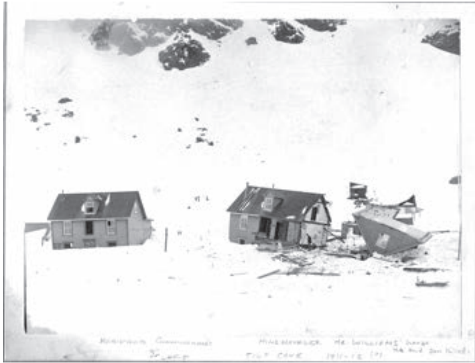
Houses destroyed in 1912 avalanche, Tilt Cove, Newfoundland.
